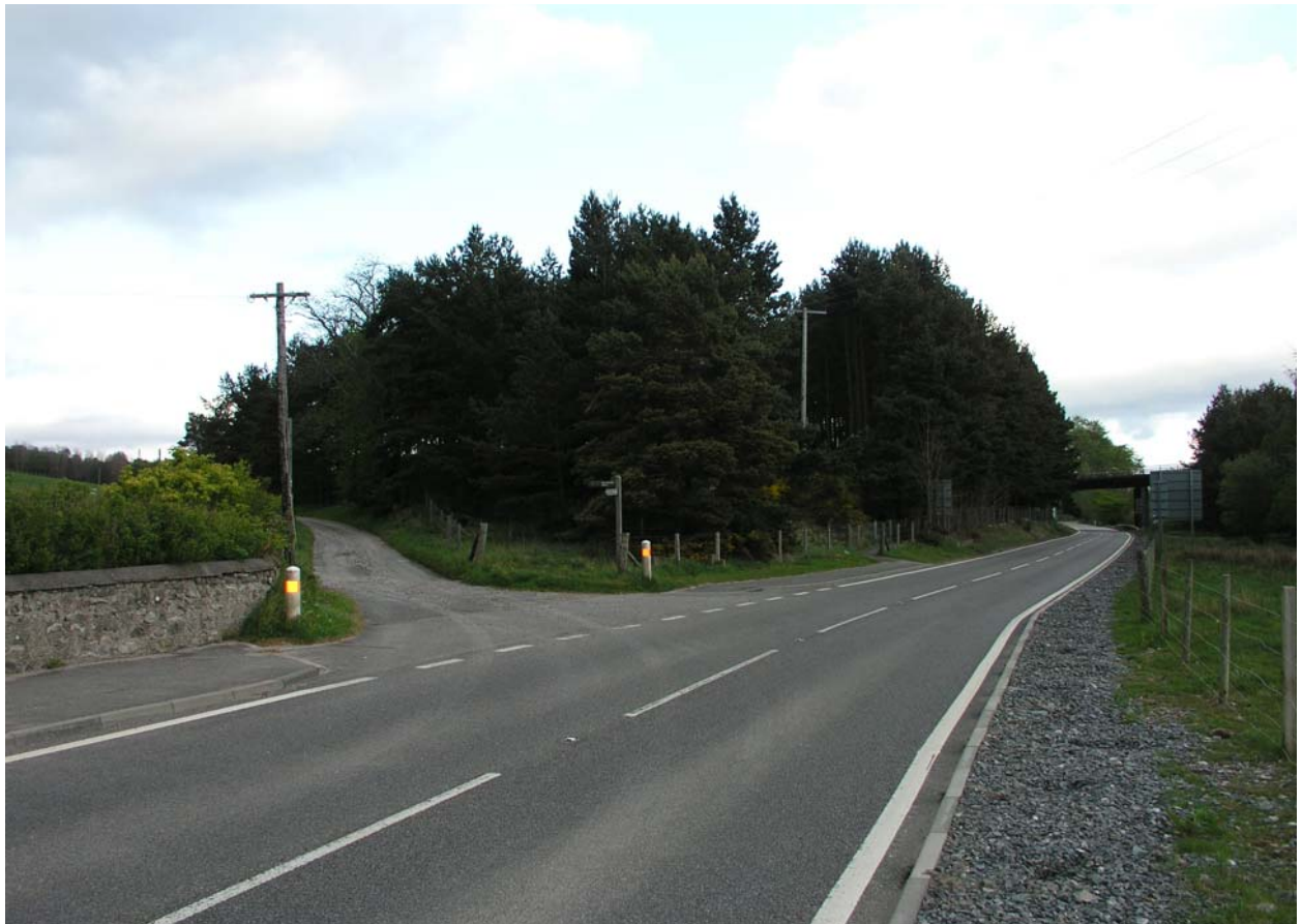
Figure 2: Photographs of current access to Kerrow Cottage from the A86
